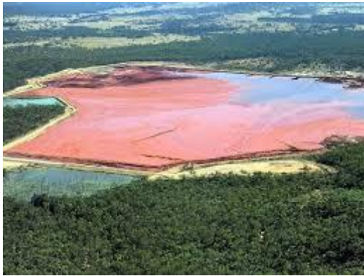
Residue disposal area
