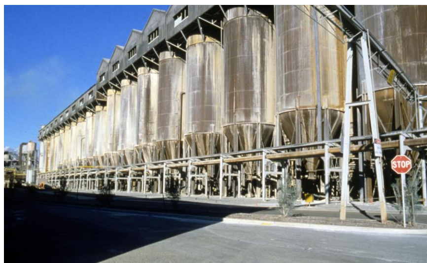
Precipitation Building with Pachuca tanks
