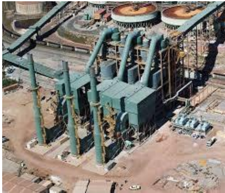
Gas suspension (fluid bed) calciners
